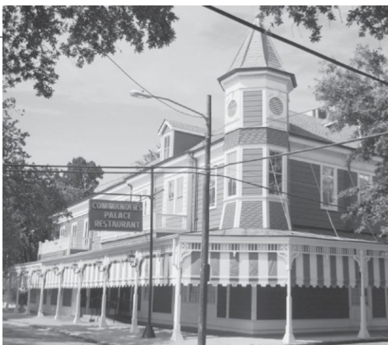
Commander's Palace. It took more than a year to repair the antebellum building after Katrina.
