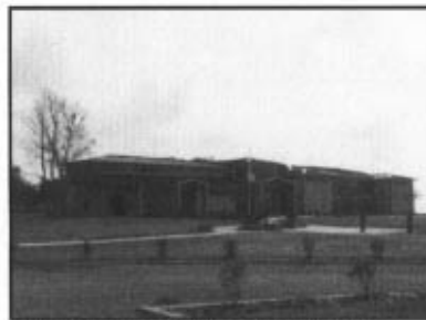
Cape Lookout National Seashore Visitor Center on Harkers Island
